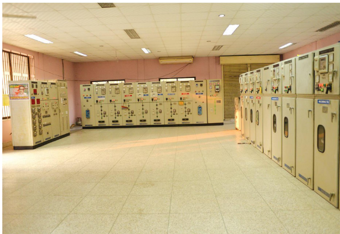
11/0.4 KV Distribution Transformer at Khulna
