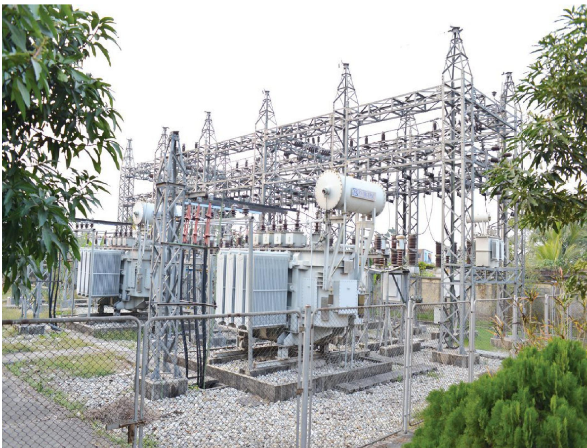
33/11 KV Substation.
